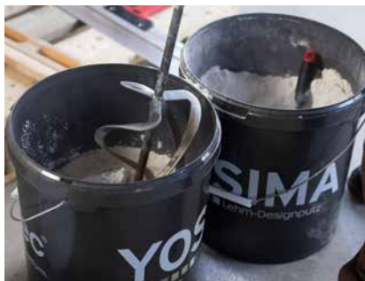
Mix the contents of the bucket into water. Let soak for 30 minutes.
