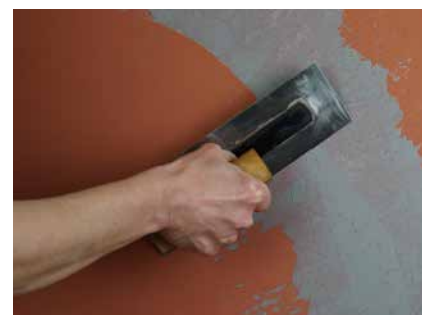
Applying the marbled topcoat
