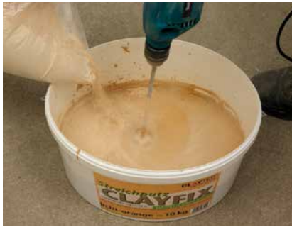
Mix bucket contents into water
