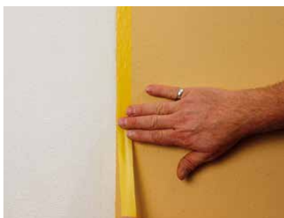
Reapplying masking tape after drying
