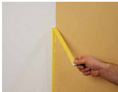
Removing the tape after wiping down
