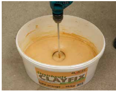
Remix thoroughly after 30 minutes of soaking
