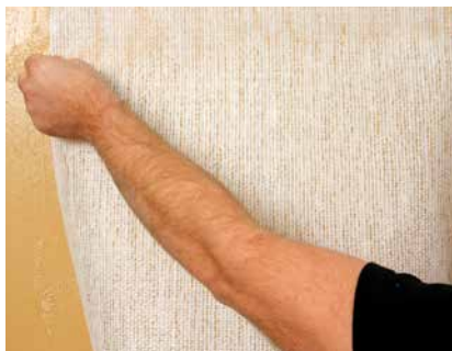
Pasting up glassfibre mesh wallpaper
