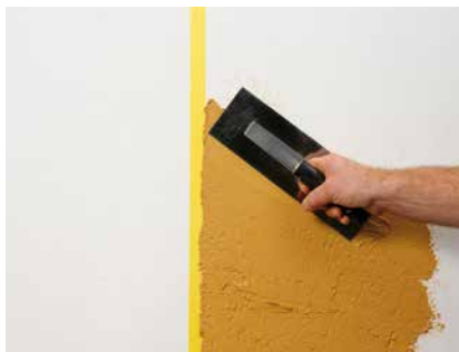
Applying the first color up to the masking tape
