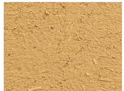
Structure of a well-prepared clay base coat surface
