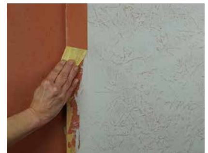
Remove at a sharp angle
