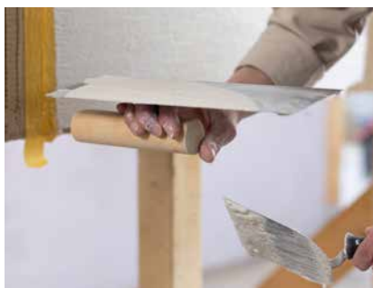
Scoop mortar from the bucket onto the trowel.
