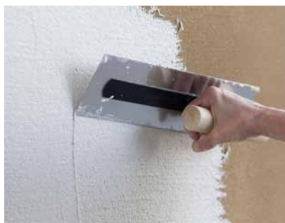
Apply mortar with the trowel.
