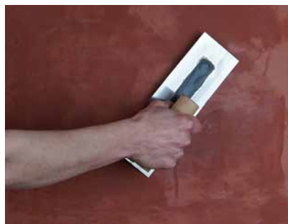
Stain filling execution
